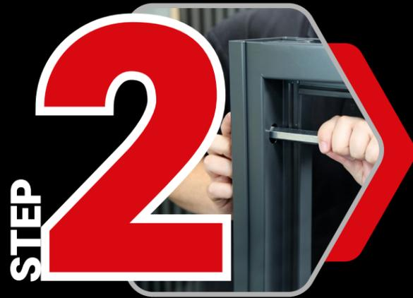
**Wind out the adjustable anchors to get the frame held in position.**
